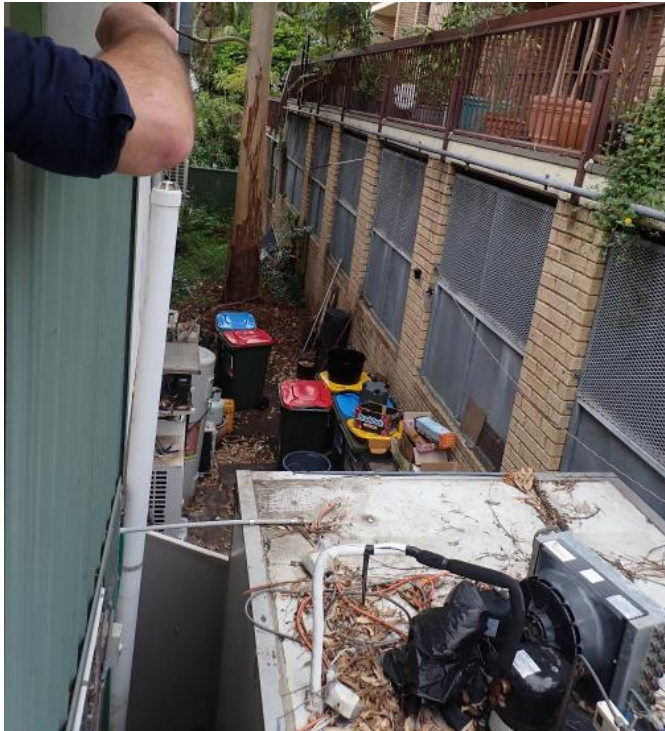
Figure 3: External view facing south showing private rear lane
