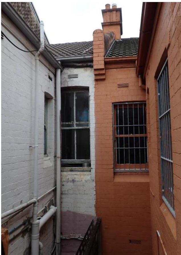
Figure 6: External view facing east showing rear wall of terrace building and party wall between 551 and 553 Crown Street
